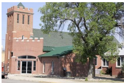
St Giles' in 2013, after renovations
